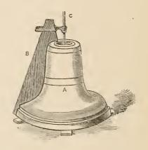
The core is hardened by a fire made in its hollow, and when it is sufficiently "set," it is covered with grease and tan, over which is placed a coating of haybands and loam, of the thickness of the intended bell, and upon this the cope or outer mould is shaped. When this is dried it is removed, the thickening of haybands and loam which represented the shape of the bell to be cast, is destroyed, and the two moulds, the core and the cope, are examined and finished.
